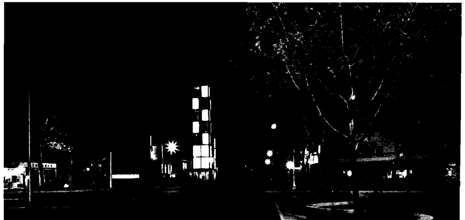
Mountain Bell's new plant addition lights up Main Street in Grand Junction, Colo.
