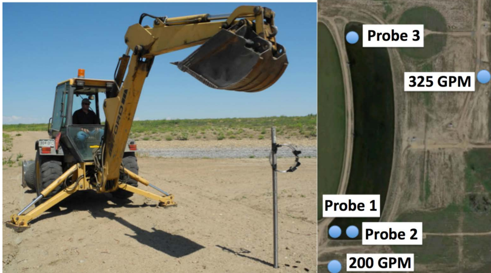
Figure 3.25: In situ high-resolution temperature sensing probe insertion with a backhoe, probe locations, and steady pumping rates during the experiment. Probe 4 was located just east of probe 3, but signal was lost due to cable breakage at some point along probe 4 possibly due to scraping a large cobble during direct push insertion.
