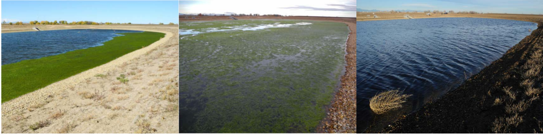
Figure 1.21: Northern view of the algae impacted eastern central infiltration pond, left (10/17/12) is the early stage of a pond flooding and algae growth, center (11/2/12) is the algae impacted stage, and right (11/22/12) shows that the algae has died and settled out.
