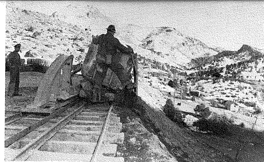
▼ Car Dump showing movable ramp.
