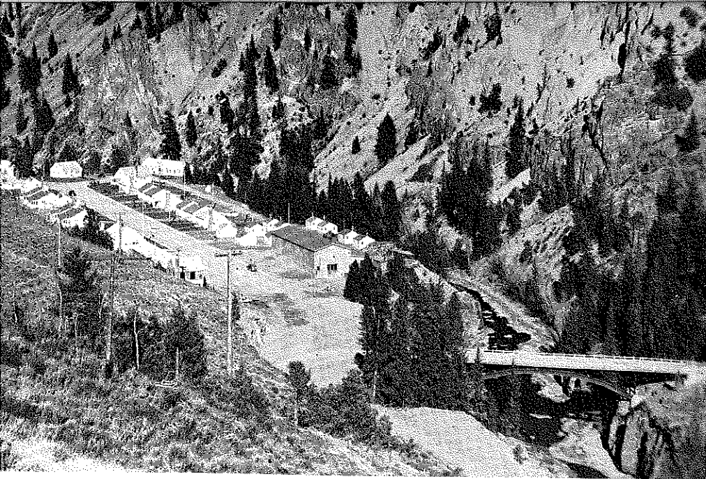
▼ Fig. 5. Government camp below Green Mountain dam. Shows Rough, craggy appearance of upper porphyry sill. Box canyon is in lower porphyry sill. Talus on slope below upper sill covers a layer of Morrison shale.
