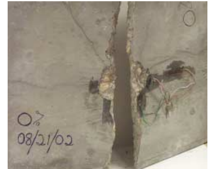
Results show conventional concrete (with 0% replacement of aggregates) after a test using one gram of plastic explosives.
