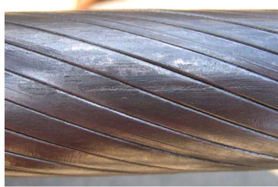
cleaned rope with visible damage
