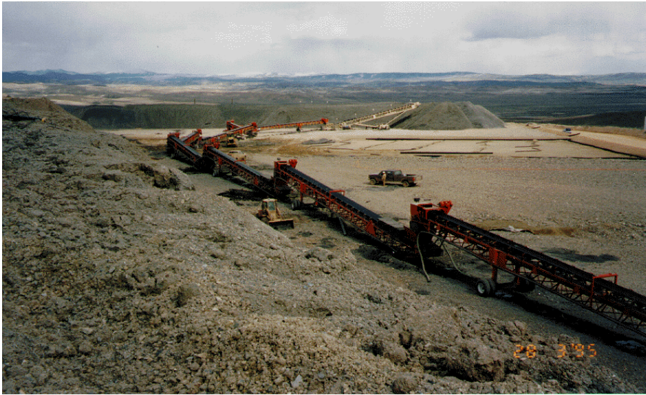
Figure 2.6. Biooxidation heap construction using conveyors (photograph courtesy of Jim Brierley, Newmont Metallurgical Services).
