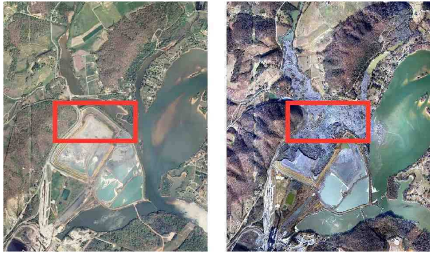
Figure 1.2: Satellite images of TVA Kingston plant and surrounding area before (left) and after (right) the failure of an earthen retaining wall. The rectangle overlaid on each image outlines the retaining wall which failed. Figure adapted from [8].
