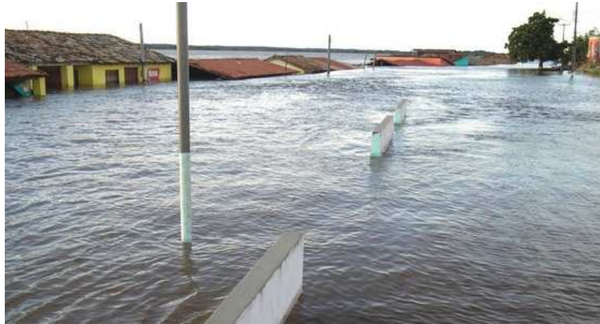
Figure 1.1: Homes washed away in the aftermath of the failure of the Algodões dam in Cocal da Estação, Brazil. Figure from [5].
