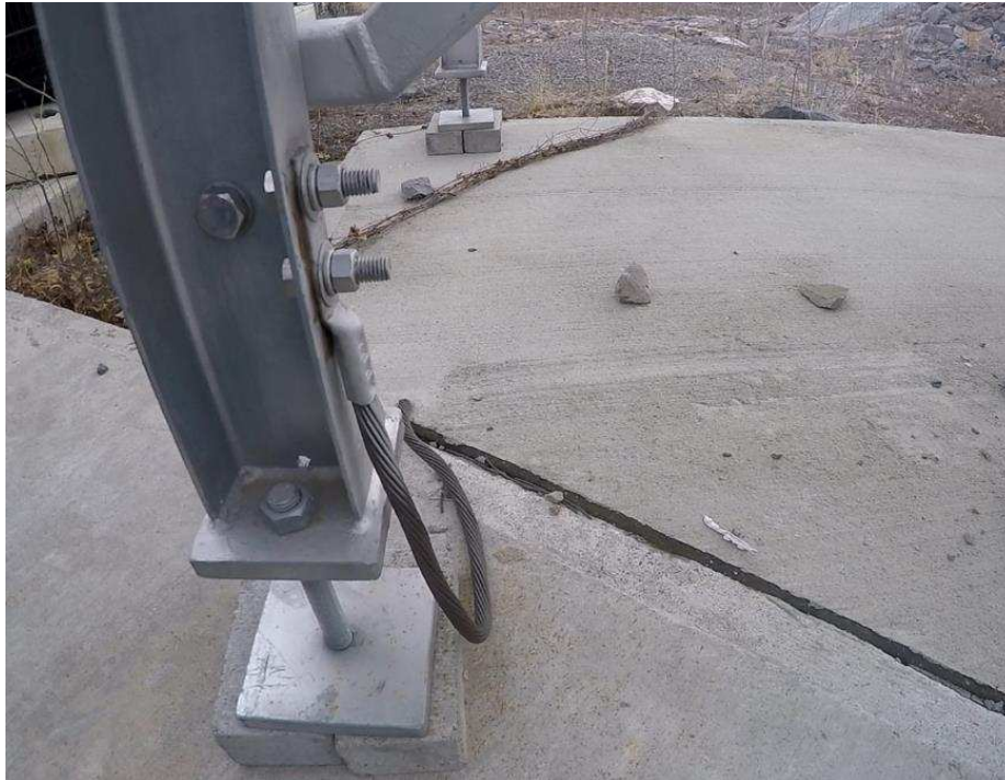
Figure 1.6 Typical Finished Grade Grounding Connection
