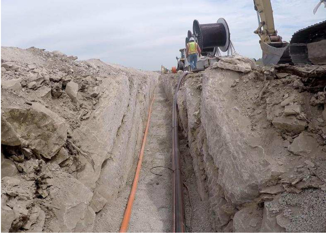
Figure 3.5 WPP Collection Trench Installation
