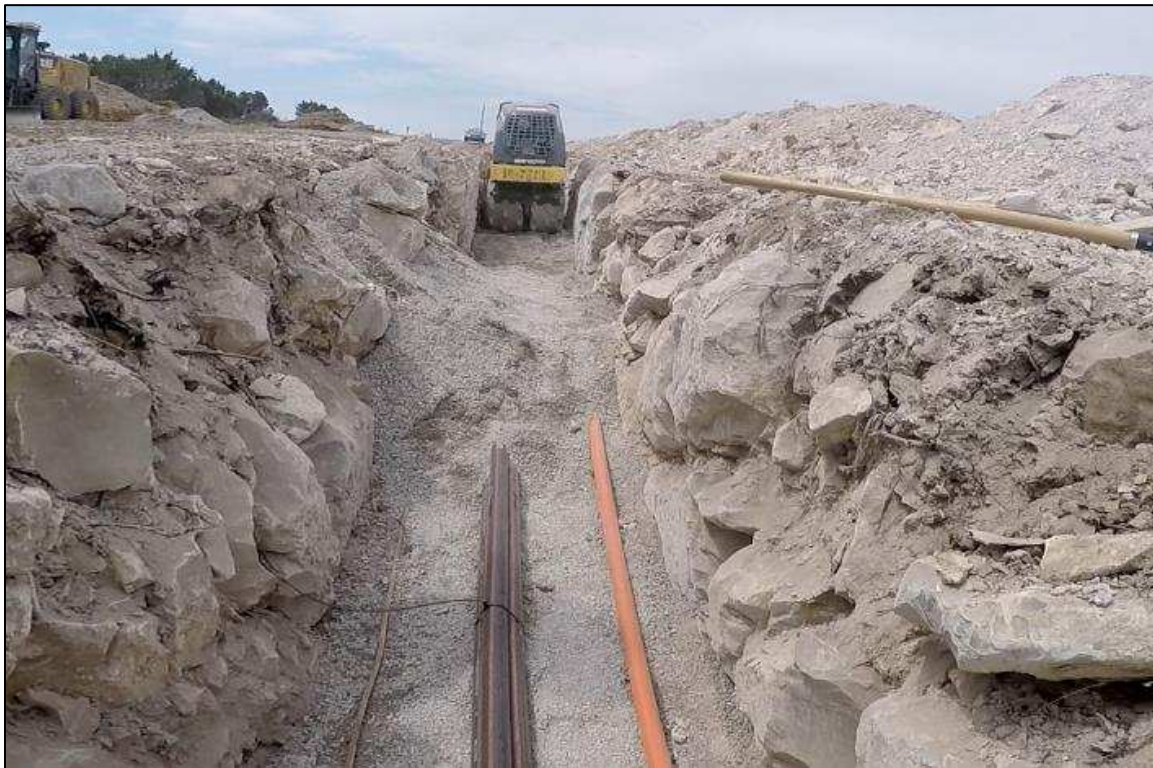
Figure 3.4 WPP Collection Trench Typical Arrangement
