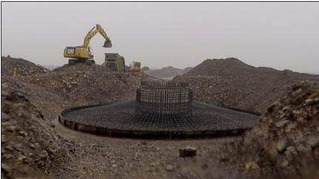
Figure 3.3 WTG Foundation Structural Steel Installation
