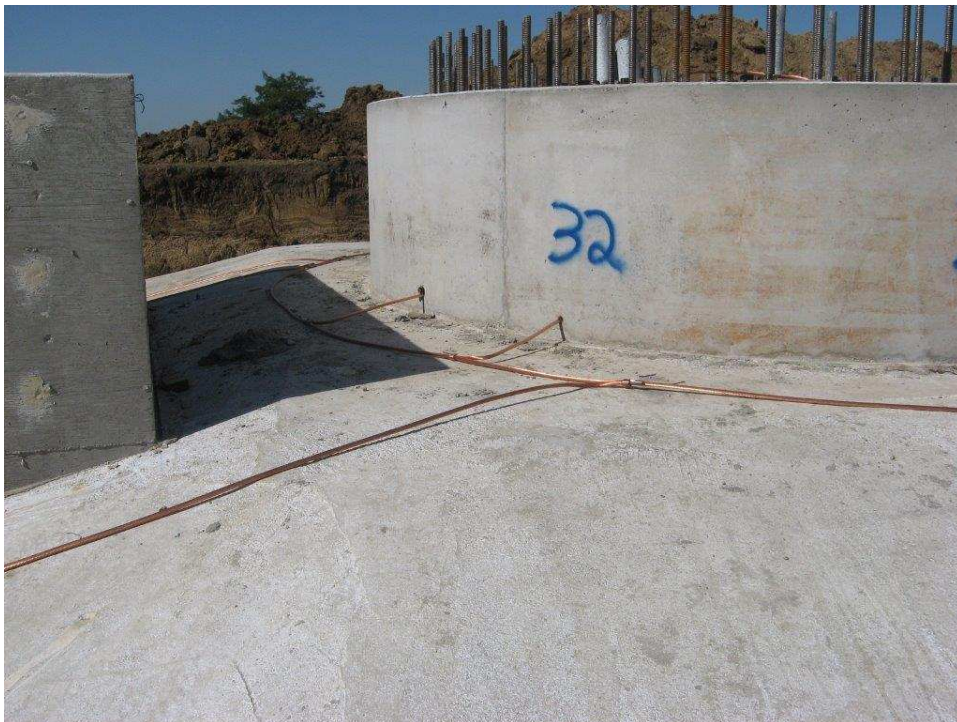
Figure 1.5 Typical Ground Grid Installation
