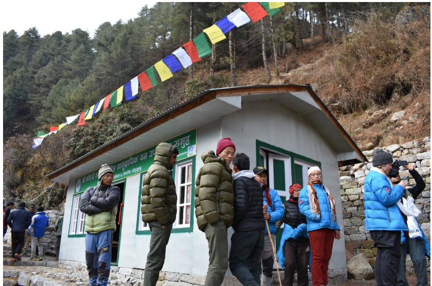
A group of local government officials and community leaders discuss the location of a new toilet with Hike for Help leaders
