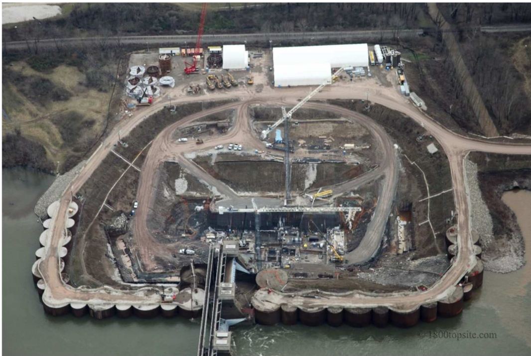
Figure 1.2. Willow Island Hydroelectric Project Cofferdam (Ciammaichella and Tantalla 2014).
