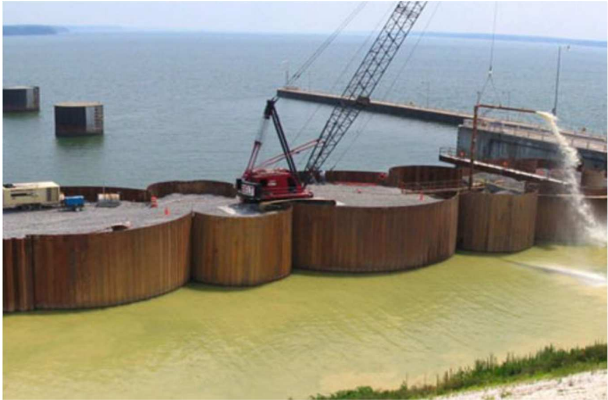
Figure 2.5. Construction of Kentucky cellular cofferdam.
