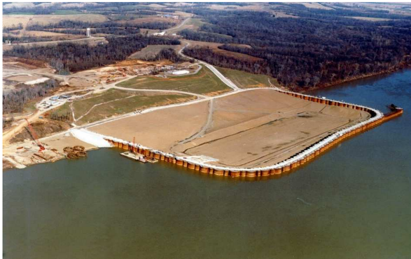
Figure 4.4. A cofferdam on the Ohio River near Olmsted, Illinois, U.S.
