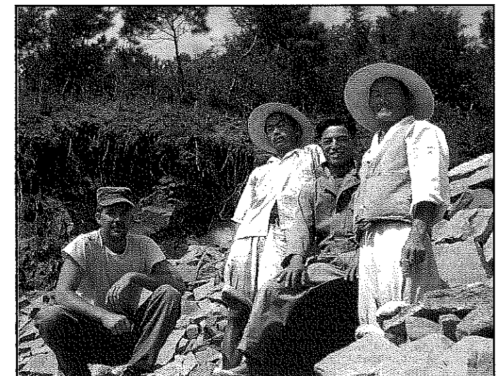
Lt. Bob "Tex" Owen '51 (left) and three Korean laborers at the Paris Mountain road construction site near Mochan, Korea in 1953.
