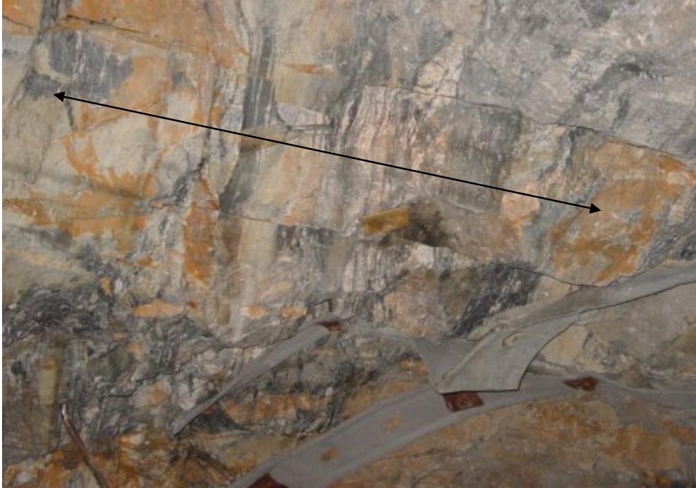
Figure 6.9 Troubling discontinuities noted before Experiment #2
