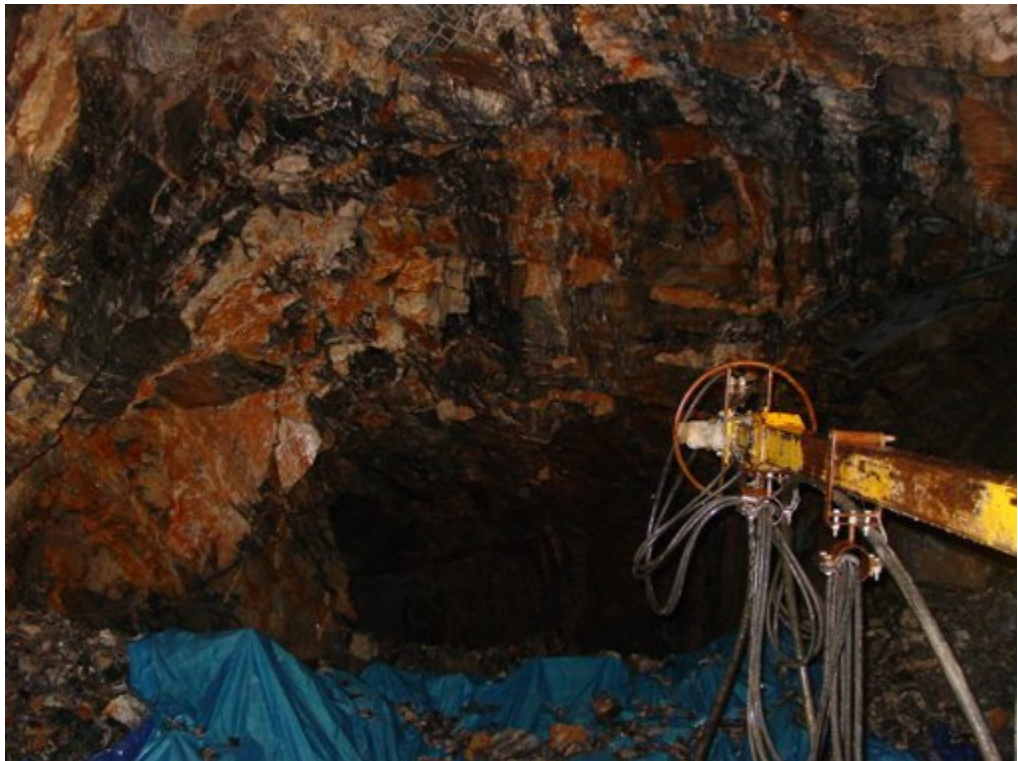
Figure 6.3 After waterjet scaling, Experiment #1
