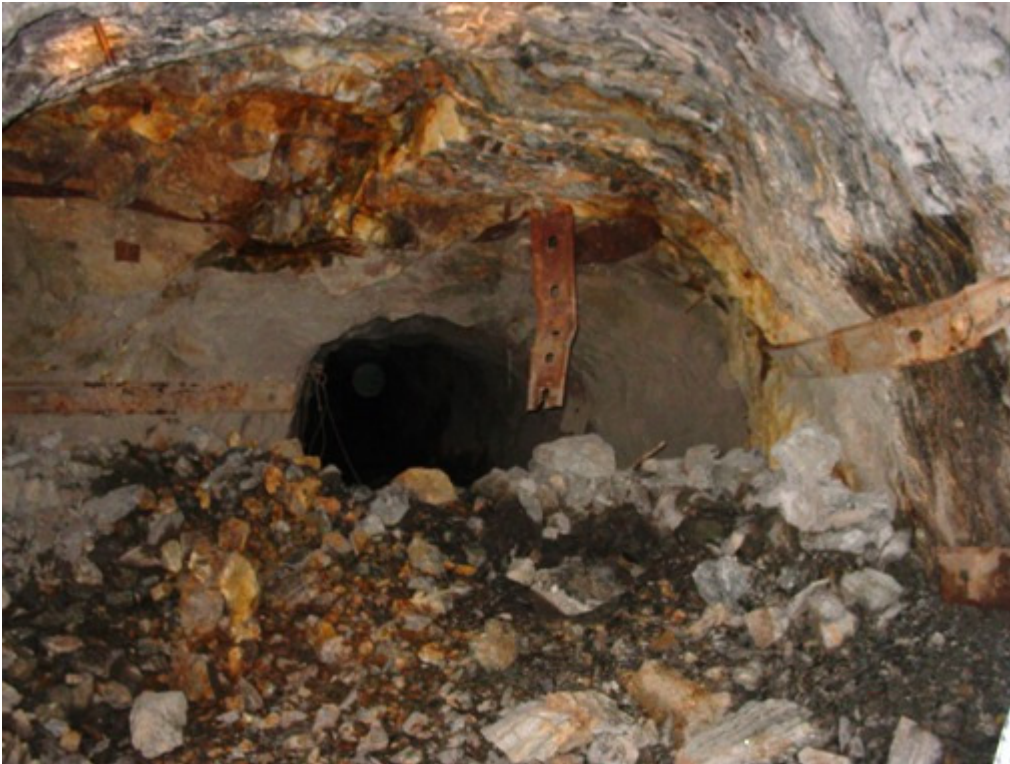
Figure 6.38 Fractured and weathered weak zone in Experiment #8
