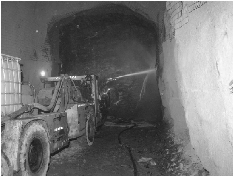
Figure 2.1 Waterjet scaling rig by MIRARCO, Sudbury, Canada
