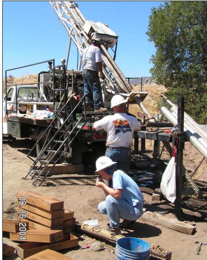
Figure 3.4: Core drilling of an angled hole DH-A.
