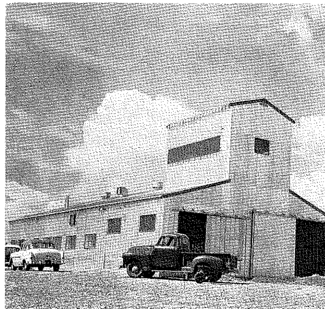
▼ Kerr-McGee Mineral Dressing Pilot Plant.
