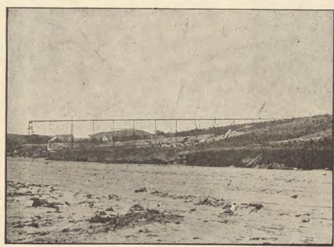
Pipe Line to Upper Pits, Where Gold Is Sluiced from the Dis-integrated Reef Matter.
