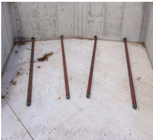
Figure 1.11: Left: Aeration tubes in the bins which must be seated to provide aeration path. Right: Drum ventilation and fan supplying moist air and gases to the aeration tubes.
