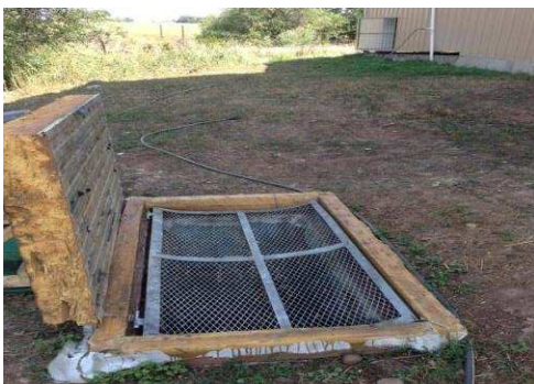
Figure 1.9: Septic tank system and screen cover
