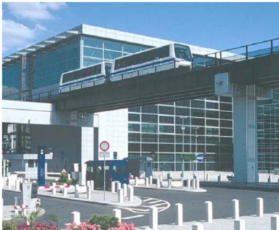
Figure 1: People Mover at the airport of Frankfurt/ Main, Germany
