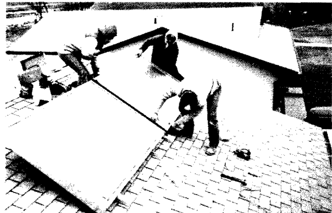
Many self-help families worked together to install solar-heating systems on their homes.
