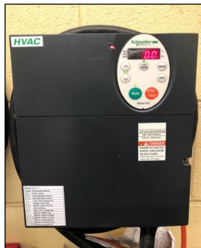
Figure 3.6: Variable frequency drive (VFD) used in the experimental apparatus.
