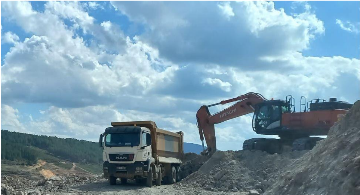
Figure 3.1 Hydraulic Backhoe Excavator Operating on a Bench Top
