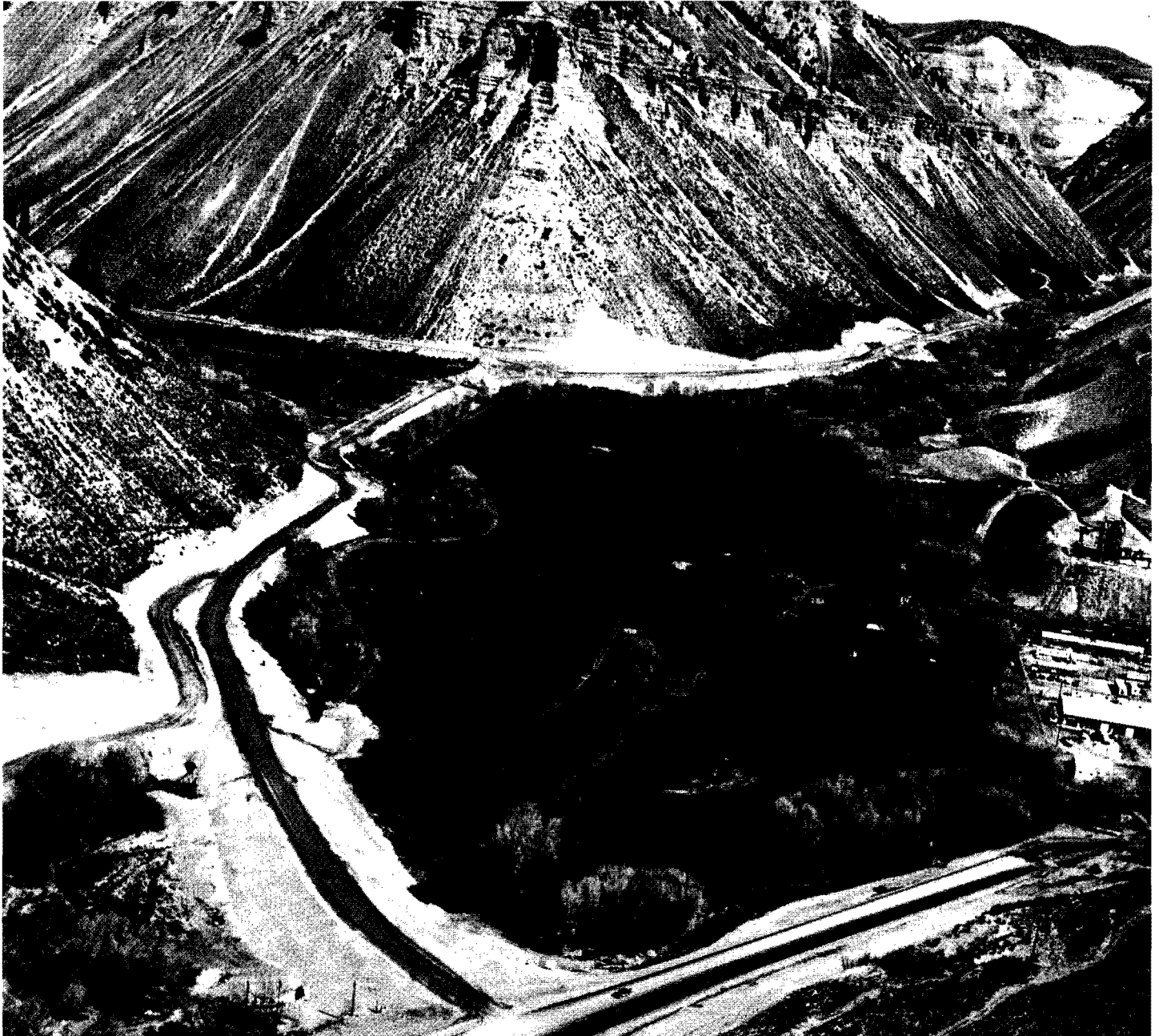
Permanent revegetation preparation has been completed along this access road at the Colony site and the slopes are ready for reseeding.
