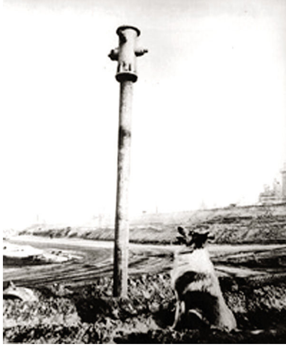
Figure 1-4. Subsidence problems at Wilmington Field in Long Beach, California. (photo courtesy of the University of Wisconsin--Stevens Point Geology Department.)
