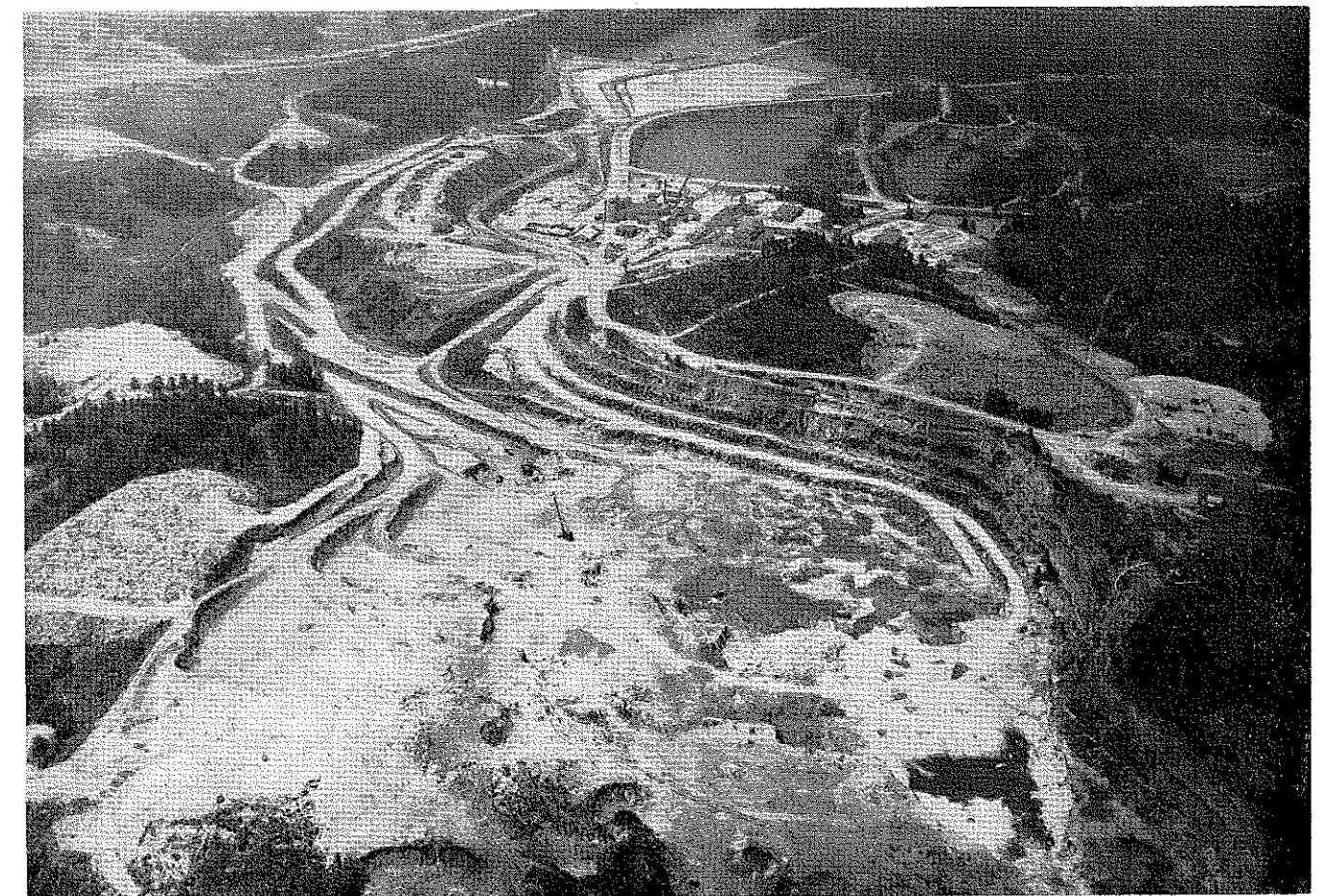
▼ Aerial view of open pit and general plant area.
