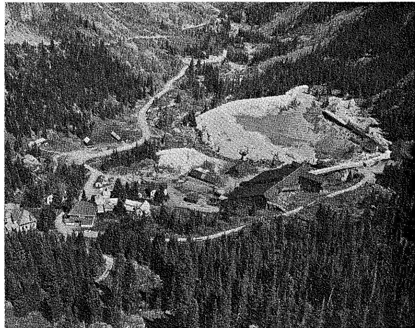
▼ A new 500-ton-per-day concentrating mill is being constructed at the famous Camp Bird mine near Ouray, Colo. The mill will be located on the site of the old mill building, shown lower right center in picture. (Photo courtesy of The Mining Record.)
