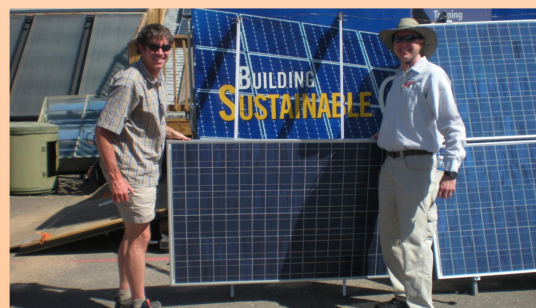
Two SEET Participants demonstrate how to install a photovoltaic panel.
