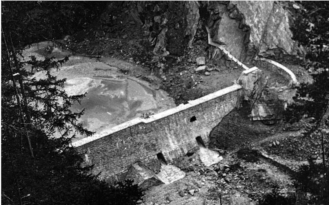
Fig. 5. Barrier with a self-cleaning function (dosing); “Strele-Sperre”, Fischbach, Längenfeld, Tyrol (IAN-Archive)
