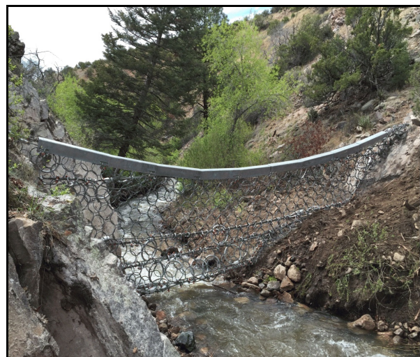
Fig 3. Post-fire VX net installed above running stream in Nambé Pueblo, New Mexico. Note basal opening allowing water and fish passage beneath. Animals can pass either underneath or through rings.
