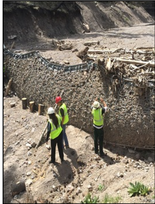
Fig 7. Filled Geobrugg UX debris net in Santa Clara Pueblo, New Mexico.
