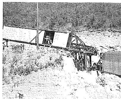
▼ View of the transfer house foundation between conveyors "A" and "B."
