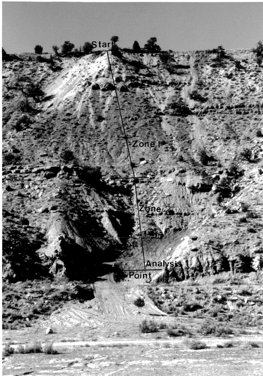
Figure 11: Slope used for CRSP testing near Rifle, Colorado.
