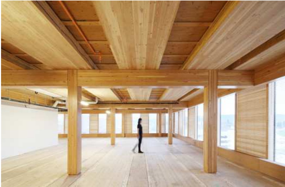
Figure 1.4: The inside of the Wood Innovation and Design Center.[9]
