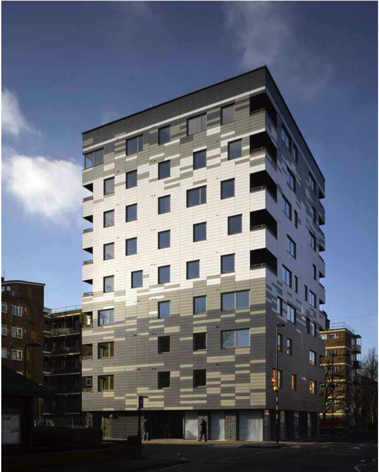
Figure 1.3: The Stadthaus building. [8]
