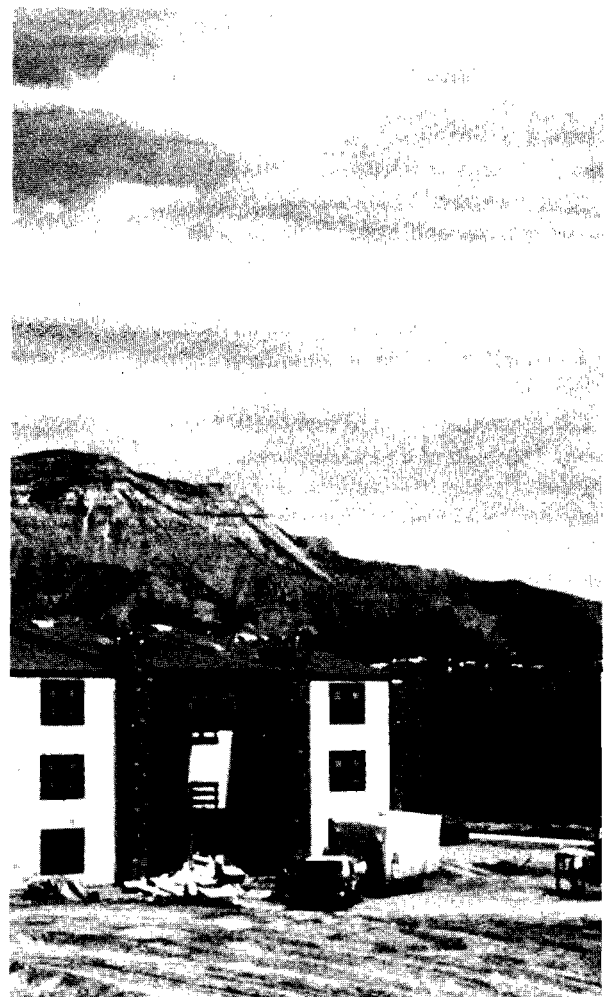
Union Oil Co. is constructing these apartments at Parachute.
