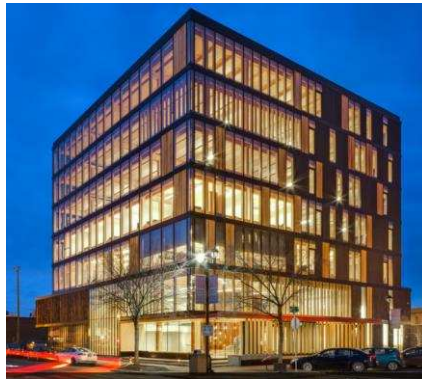
Figure 1.2: Wood Innovations and Design Center [17]
