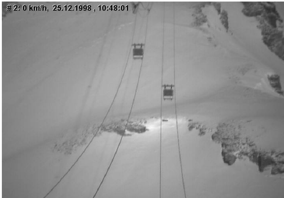
Figure 16 Image from the video camera mounted on no. 2 tower of the Funitel in Montana
