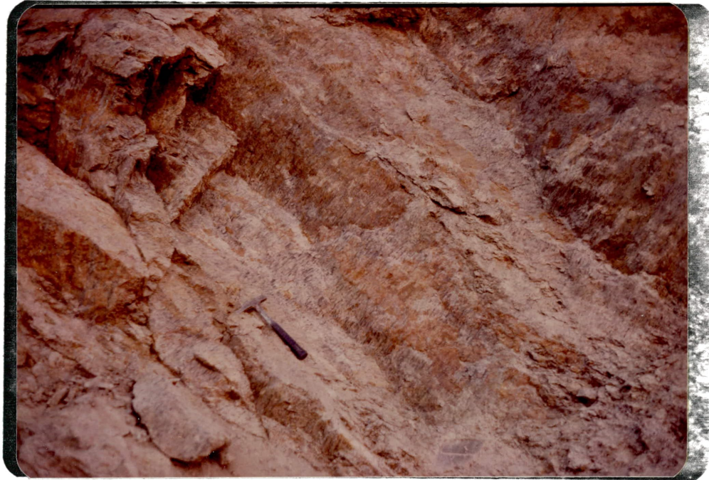
Figure 109. Uniformly oriented slickensides in the serpentine zone (east wall). Looking to the east.
