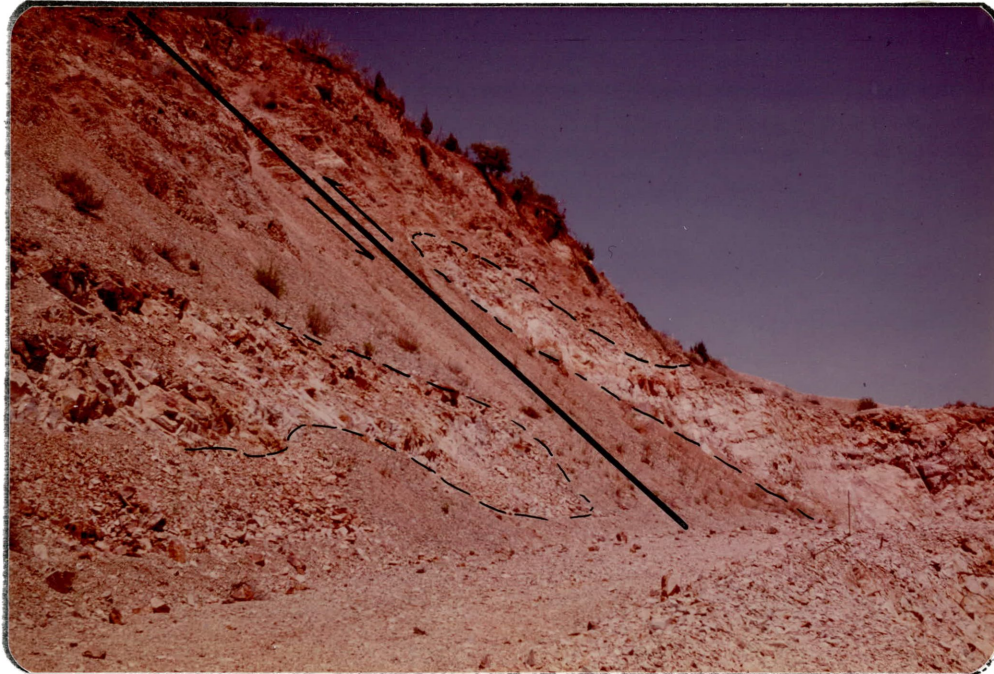
Figure 92. Highly weathered hornfels (Colorado Shale). Location: upper west and northwest walls of the pit. Notice the displacement of the Beartooth Quartzite (the resistant bed) by the fault.
