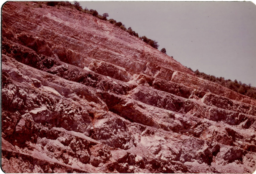
Figure 119. Major fault and minor fractures with intensive oxidation along the fracture planes due to water seep. Location: southwest wall.
