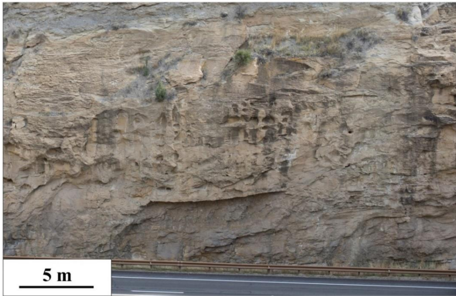
Figure 2.10 The exposed massive sandstone at the southern part of Site 2. Photo courtesy CDOT.
