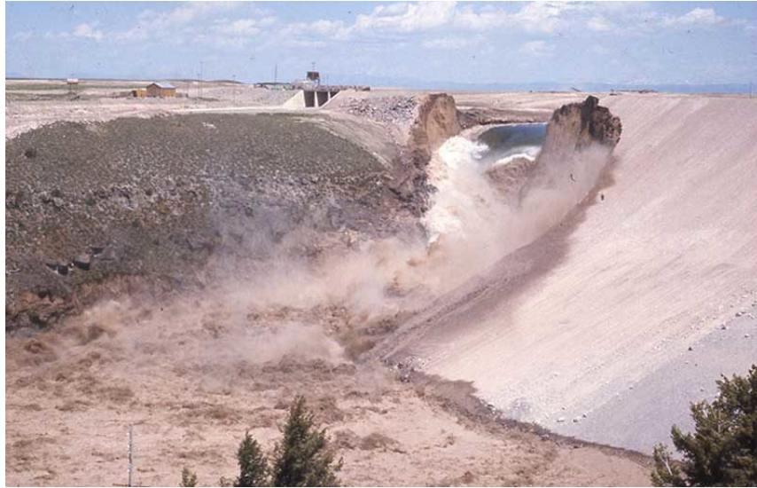
Figure 1.1. Photograph of the Teton Dam failure near Rexburg, Idaho in 1977 (USBR, 2020).
