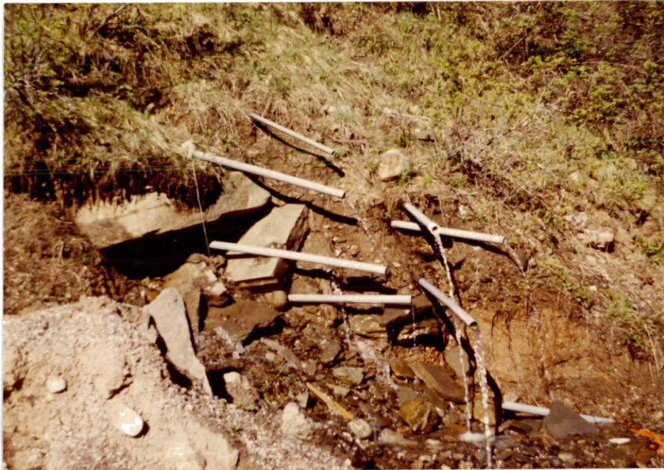
Figure 24. Horizontal drains used on the Whiskey Creek Landslide, north of Minturn.
