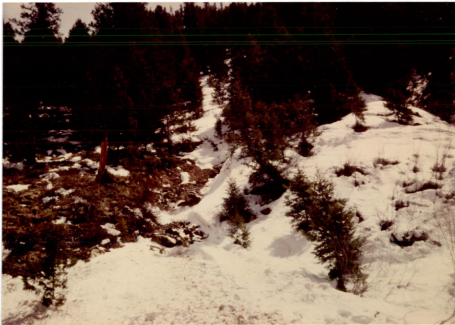
Figure 14. Drainage above TH-9 running directly into the slide. Note snow avalanche debris in the foreground.
