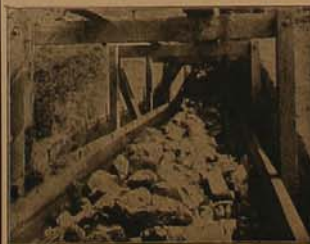
Coal Conveyor, 328 ft. center handling 4 tons run of mine coal per minute
