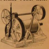
Is light and portable weighing 1050 lbs., heaviest piece weighs 150 lbs., capacity 1000 lbs. one hundred foot per minute, will lift 400 feet. A Safety latch follows every foot of the lift, guaranteeing absolute safety.
