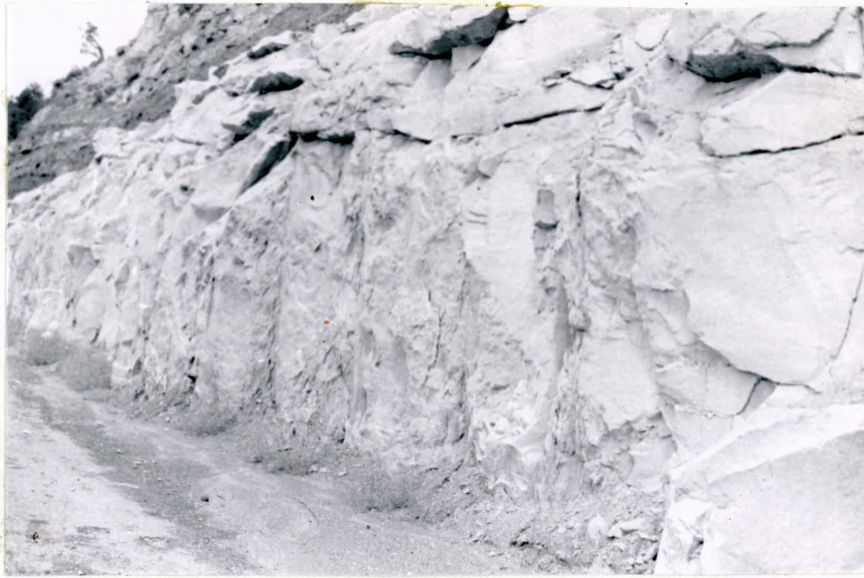
Figure 49. The massive sandstones of the Raton area are fractured by several joint systems. Railroad Canyon.
