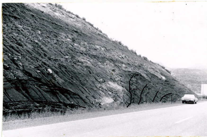
Figure 27. Unit No. 3, Raton Formation. Depression of underlying strata as a result of deposition of large sandstone boulders. Penecontemporaneous compression. Interstate Highway 25.
