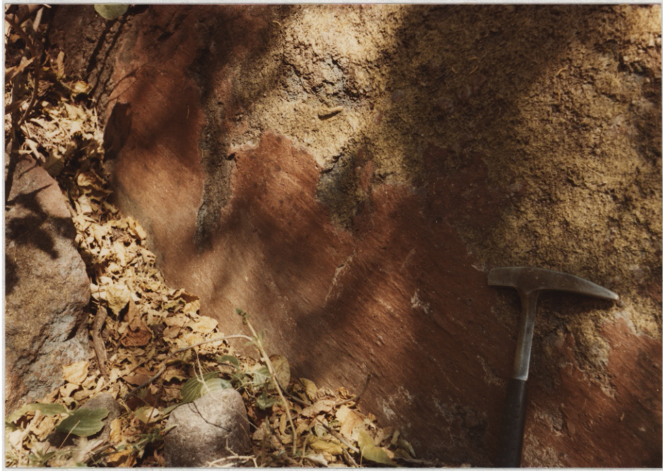
Figure 18. A post-ore fault outcrop, cutting the Huautla Complex-Early Dacite Flows, 300 m west of the Santiago mine shaft. The slickensided, hematite-rich fault plane is typical of the post-ore faults. The moderate propylitic alteration visible in the wall rock results from the nearby Santiago vein.
